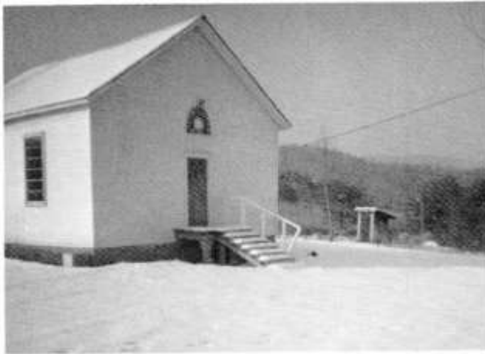
The Coulterville Baptist Church, shown in a late 1950's photograph, was originally the black school up the hollow. In the early 1930's it was moved over a half a mile to its present location where it has been renovated several times. Another sign of that time period is pictured in the yard - the outside toilet.
