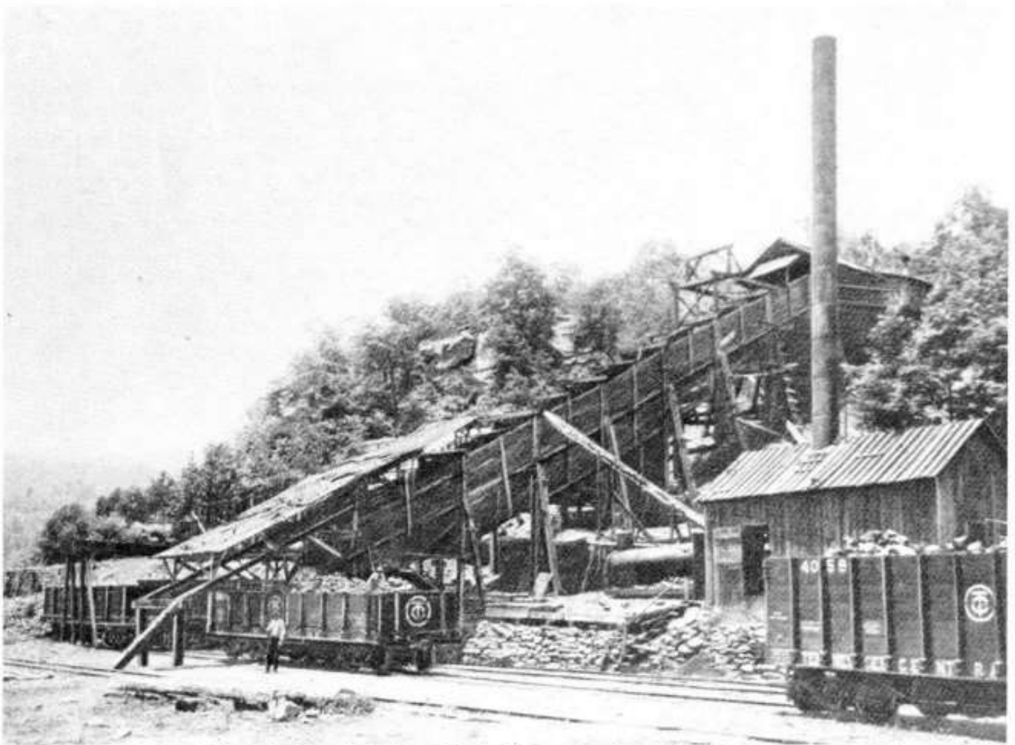
The coal tippie of the Sale Creek Coal and Coke Company, shown here in a photograph taken in 1900, was located at the foot of Sale Creek Mountain approximately one-quarter mile below the hair pin curve at the foot of the mountain. It was capable of loading 400 tons of coal daily. The smoke stack is most likely part of the steam generating system that operated the conveyors on the chute.
